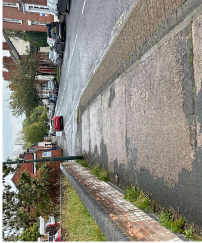
Figure 18 Uneven footways create an uncomfortable environment for wheeling
